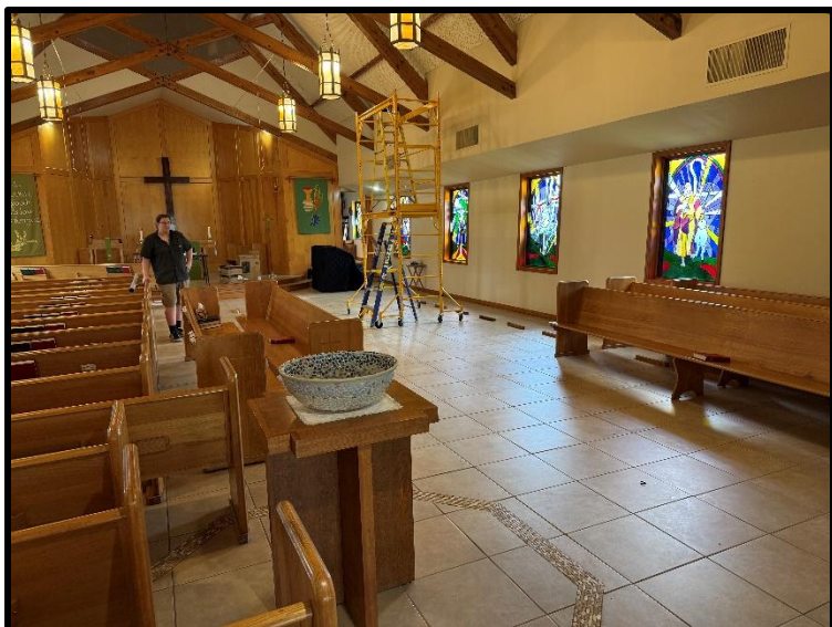
Moving the pews for the scaffolding!
